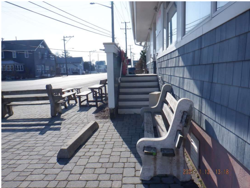
Figure 4: Front Steps Leading into Existing Building
