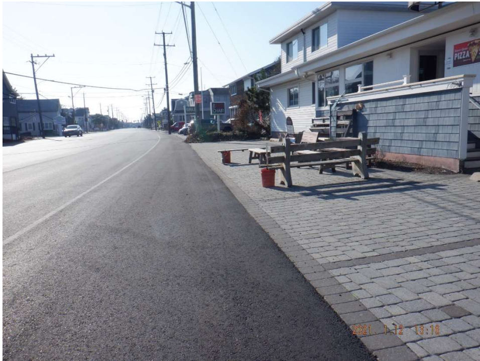
Figure 3: View of Road Infront of Existing Building
